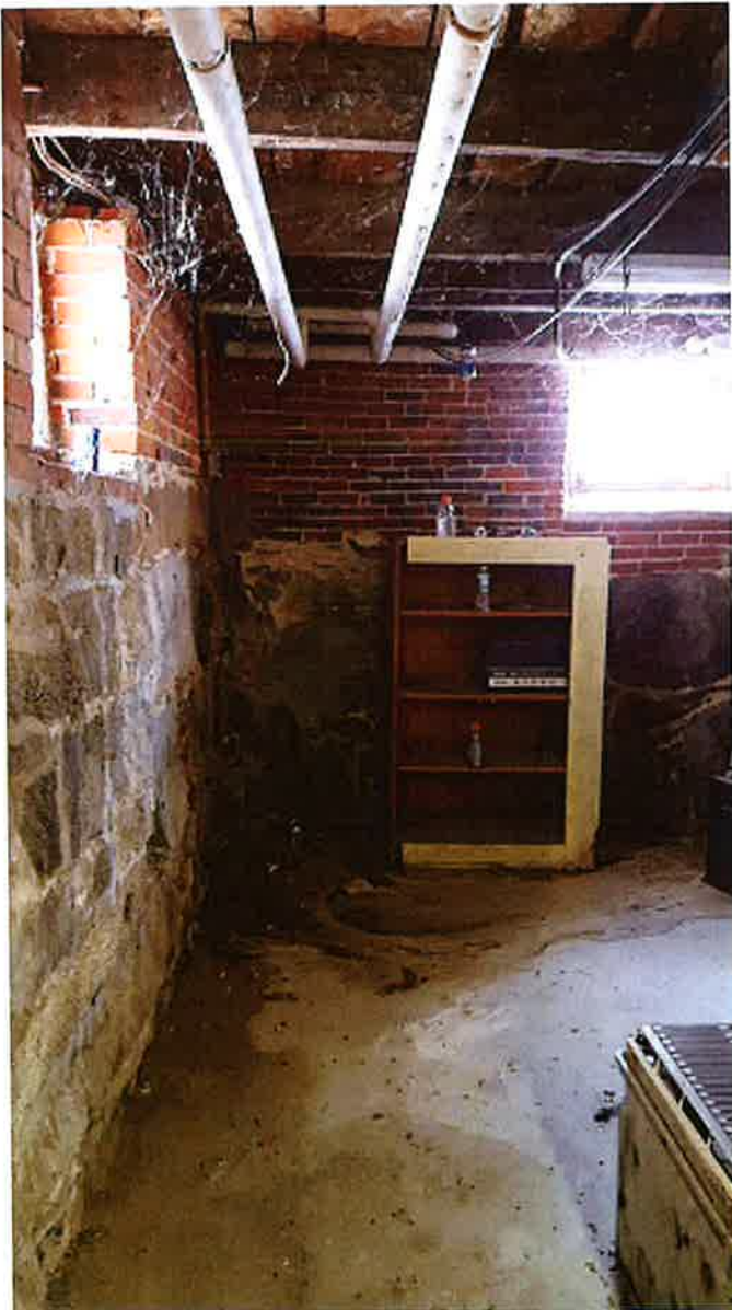
IMAGE 7 - 8 GILMAN LANE BASEMENT
