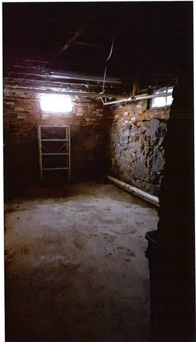
IMAGE 8 - 8 GILMAN LANE BASEMENT
