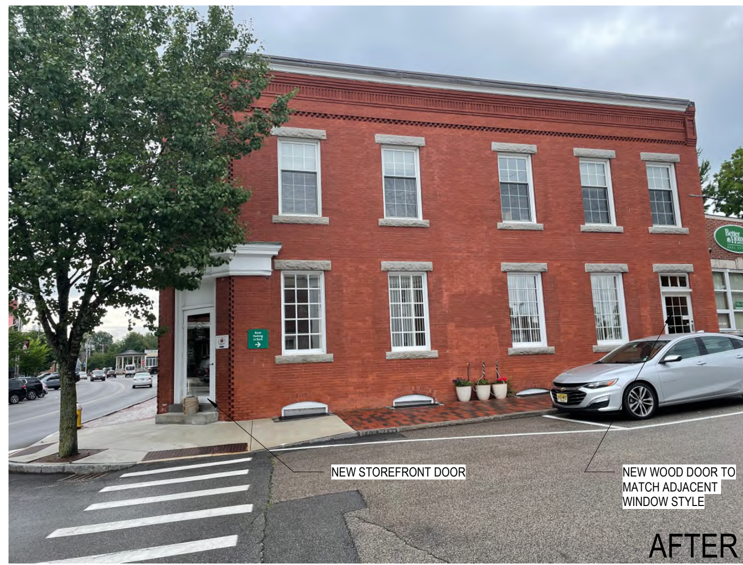
PROPOSED NEW WHITE STOREFRONT DOOR (LEFT) AND NEW DOOR WITH TRANSOM AND MULLIONS TO MATCH EXISTING WOOD WINDOWS TO REMAIN (RIGHT), REUSE WOOD DOOR FROM WATER STREET IF POSSIBLE - VIEW FROM CENTER STREET
