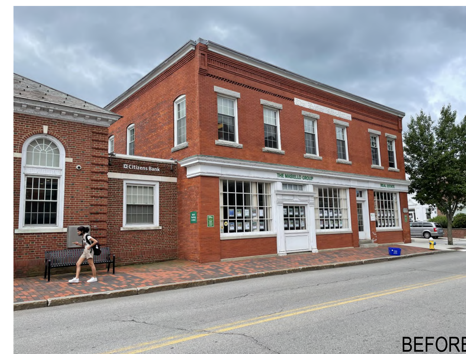
EXISTING WOOD WINDOWS - VIEW FROM WATER STREET
