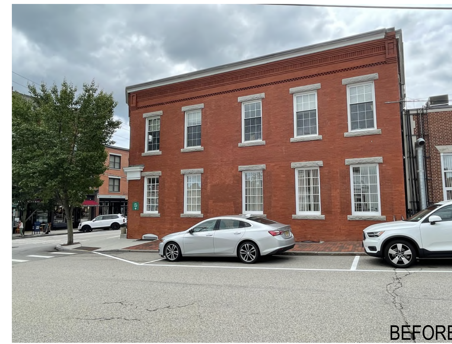
EXISTING WOOD WINDOWS - VIEW FROM CENTER STREET
