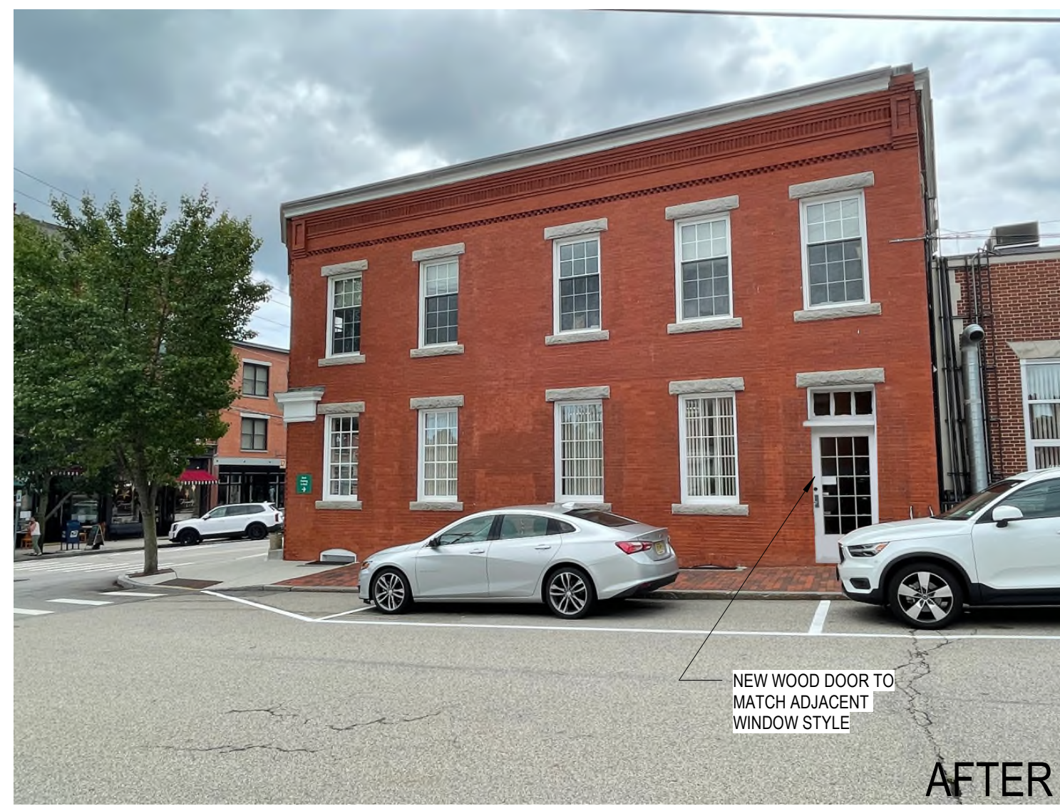
PROPOSED NEW DOOR WITH TRANSOM AND MULLIONS (RIGHT) TO MATCH EXISTING WOOD WINDOWS TO REMAIN REUSE WOOD DOOR FROM WATER STREET IF POSSIBLE - VIEW FROM CENTER STREET
