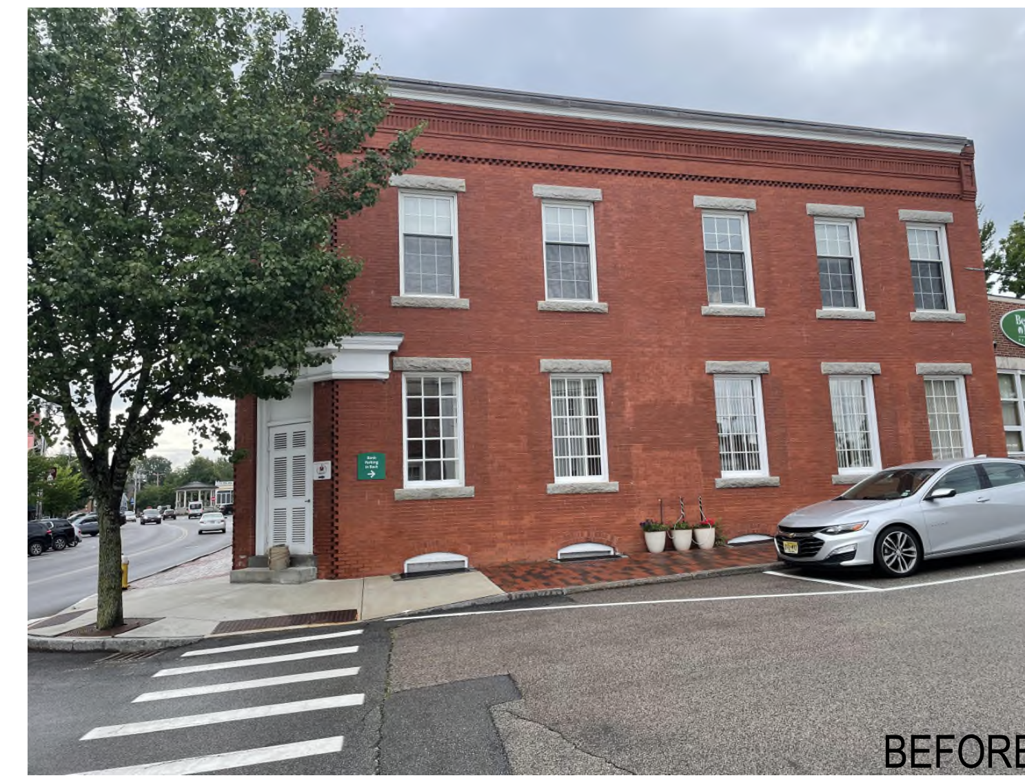
EXISTING WOOD WINDOWS - VIEW FROM CENTER STREET
