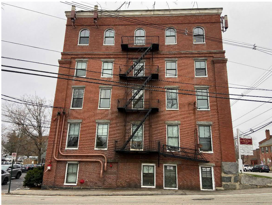
Photo 4 View of the site facing west
