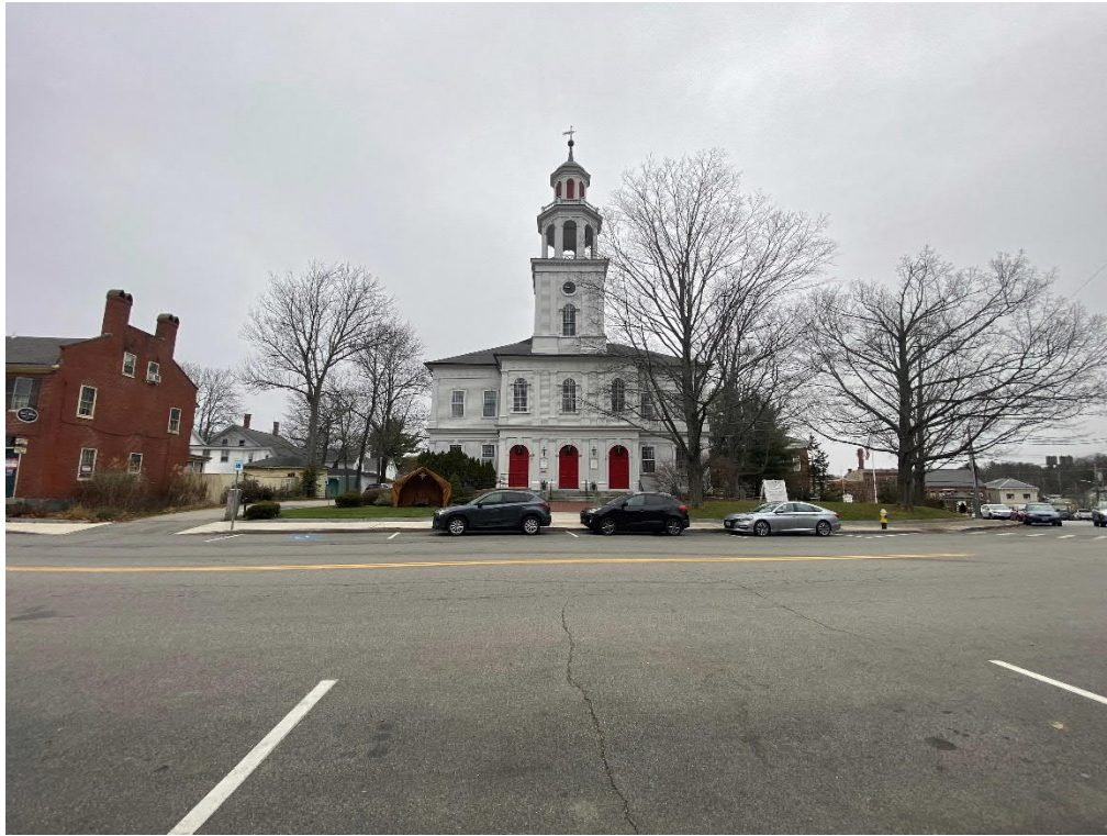
Photo 5 View from the site facing north at Front Church (NRHP Listed)
