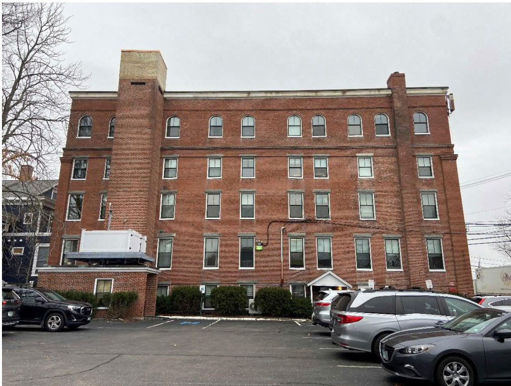
Photo 1 View of the site facing north
