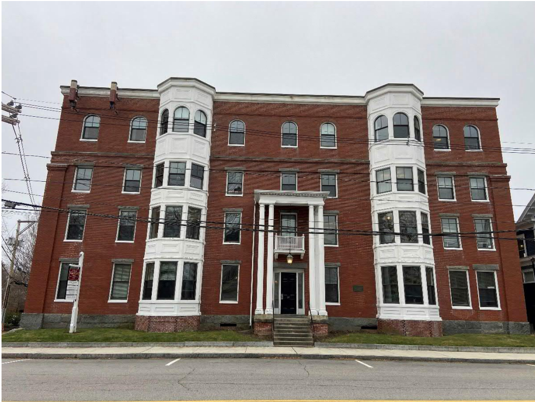
Photo 3 View of the site facing south
