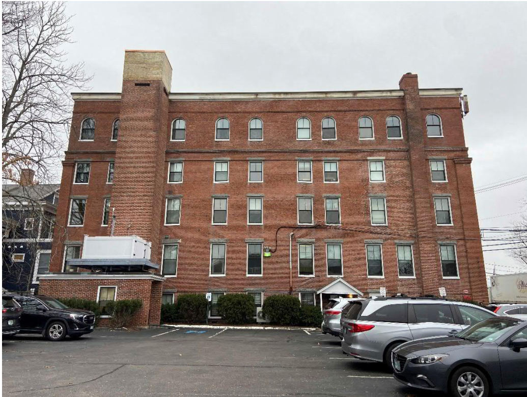
Photo 1 View of the site facing north
