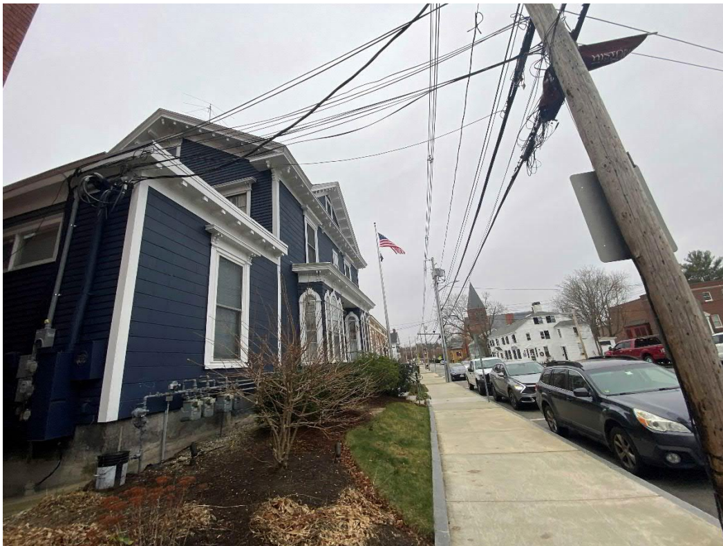
Photo 8 View from the site facing west
