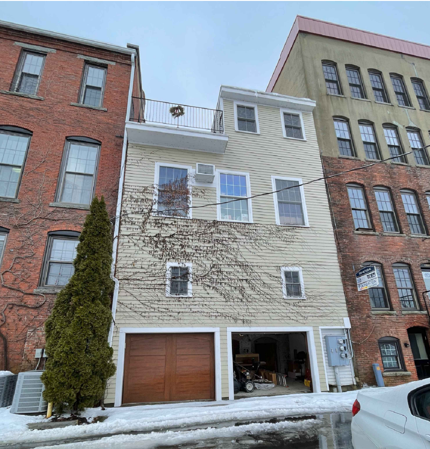
2 EXISTING CONDITIONS PHOTO SCALE: NONE
