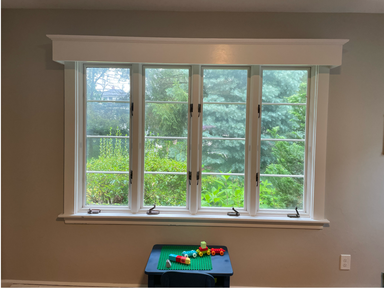
Current front window - left side of house when facing from the street:
