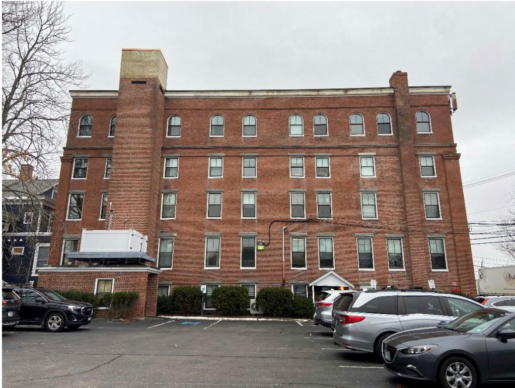
Photo 1 View of the site facing north
