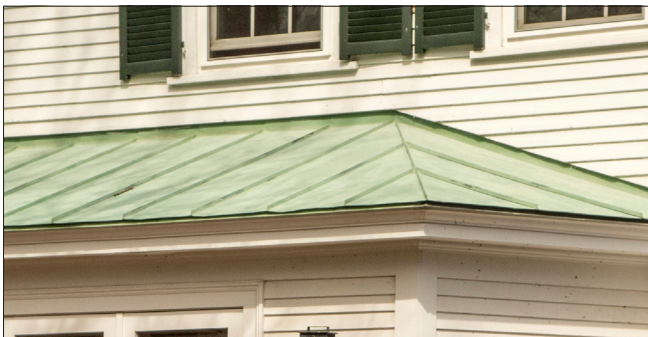
Copper is a traditional metal roofing material that does not require painting. The standing seams, as shown in this example, create a regular pattern along the roof surface.
