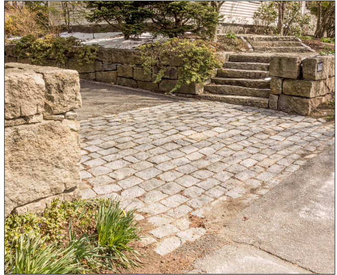
The stone retaining wall includes integral steps and the driveway has a cobblestones along the sidewalk enhancing the historic character.
