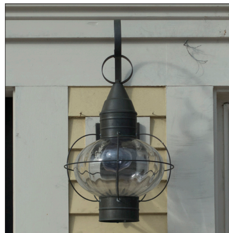
Lighting should be compatible with the architectural style of a building. It should be installed in a manner that illuminates the needed areas, such as next to an entrance door, while minimizing spillover onto adjacent properties or into the night sky.
