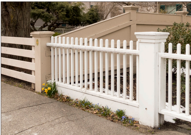
Picket and horizontal board fences are located along the sidewalk, while a solid wood fence between the properties provides privacy, tapering down towards the street.
