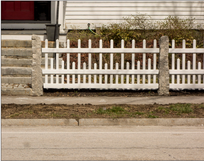
The wood picket fence is supported by granite piers.
