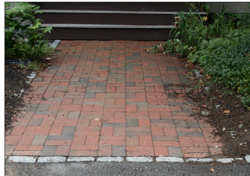
This brick walkway has a cobblestone border providing a formal entrance using traditional materials.
