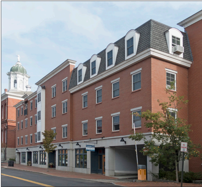
New commercial buildings should include a defined storefront with larger windows with punched double-hung and casement windows on upper floors.
