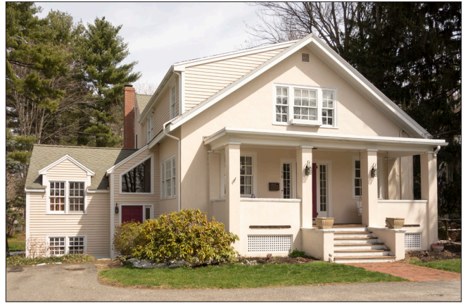
The new addition, located towards the rear, is both compatible with the historic house and contemporary in design. The smaller massing clearly identifies the addition as a secondary building volume, and both the materials and windows are compatible with the historic house.
