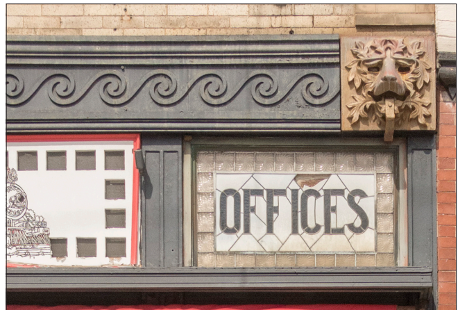
Storefront cornices can be highly decorative and serve to separate the storefront from the building above.
