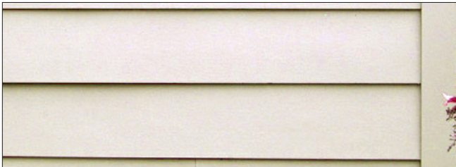
Fiber-cement siding and trim generally does not have the same dimensions as traditional wood elements including the width of corner boards and the depth of individual clapboards. This results in visual differences when compared to wood siding.
