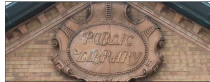
Terra Cotta - A fired-clay, non-structural building component; used for ornate details.
