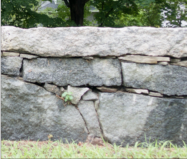
Granite, which is readily available in Exeter, is a very durable material that is ideal for the construction of landscape walls. This dry-laid granite wall includes larger stones held in place by smaller ones, all topped by a relatively flat capstone.
