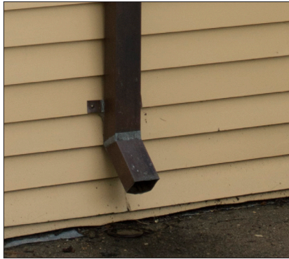
This rectangular copper downspout discharges stormwater away from the building foundation.
