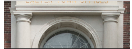
Limestone - A sedimentary rock; used for building walls, window sills and lintels, ornamental stone trim and sculpture.
