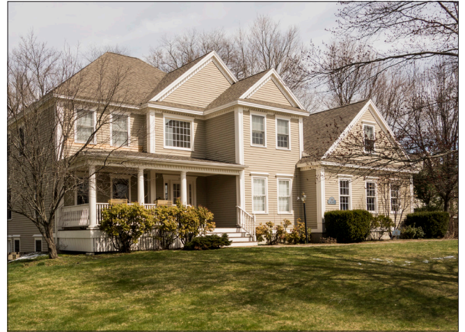
This house is sited in a manner similar to its neighbors. The multiple gable and hipped roof break down the overall mass and scale to be similar to its neighbors. The fenestration pattern includes punched window openings, avoiding a front-facing garage door.
