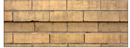
Yellow Brick - A hard, dense, fired-clay, regularly shaped building component made from high lime content clay.
