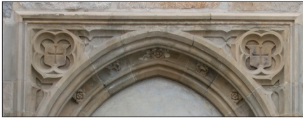
Sandstone - A sedimentary stone used as a building material, popular in the late 19th century.
