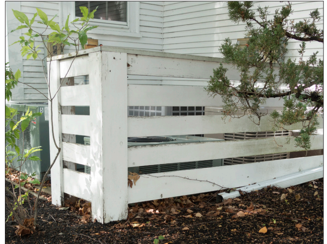
Ground mounted equipment can often be screened with fencing or shrubs to minimize its visibility.
