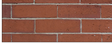
20th Century Brick - A hard, dense, fired-clay, regularly shaped building component; sometimes with a glazed surface.
