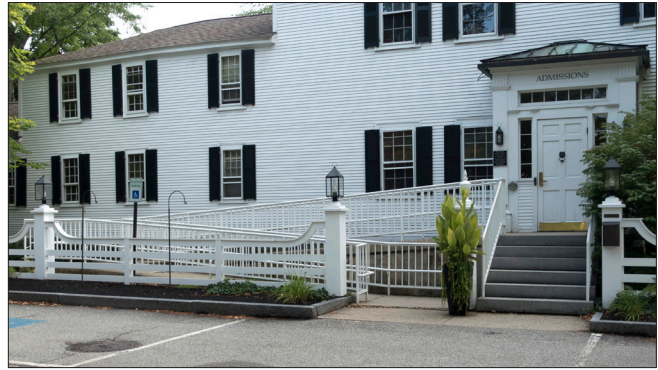
The accessible ramp allows all visitors to enter through the same door while maintaining the stair configuration.
