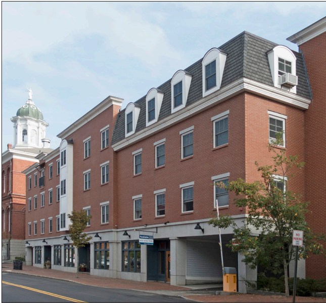
New commercial buildings should include a defined storefront with larger windows with punched double-hung and casement windows on upper floors.
