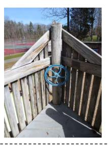
Is there a minimum of 32" access? No Less than 32" clear. Has the fault been repaired? No Is there a minimum of 17" clear under the steering wheel to the wall it is mounted on? Less than 17" Has the fault been repaired? No Is there 24" clear from safety surface to bottom of Yes steering wheel?
