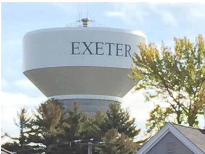
Exeter Water Tower
