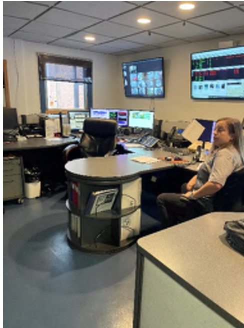
Figure 7 - Two of Three Dispatch Workstations.
