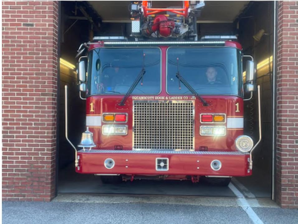
Figure 54 – Limited Clearance – this image demonstrates a lack of appropriate apparatus clearance which can complicate response and create difficult conditions to operate vehicles. This has already resulted in multiple incidents including one accident that caused $27,000 in damage and placed the aerial ladder out of service for an extended period.
