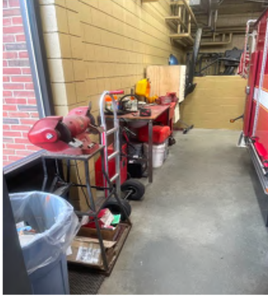
Figure 13 – Adapted Space - Adapted tool and maintenance are on the sides of the station. This presents an operational issue as well as the inability to properly store and secure vital tools.
