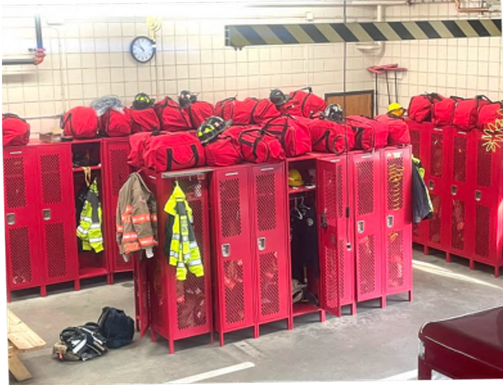
Figure 9 – Personal protective Equipment Improper Storage - Turnout Gear storage in the apparatus bays decreases the useable space for apparatus, lacks particulate separation, proper ventilation, climate control or protection from UV light which deteriorates the components of turnout gear.
