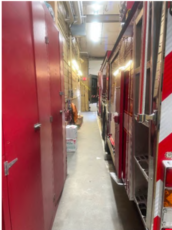
Figure 14 – Limited Space and Clearance – this image clearly shows the space limitations that have emerged as the size of apparatus has increased.
