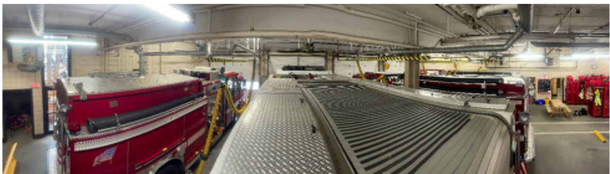
Figure 910– Lack of Clearance – Operational Inefficiency - Low ceiling height prevents easy hose loading or filling engines with water.
