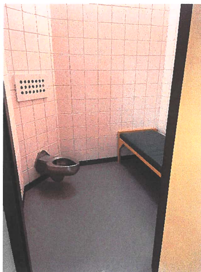
Temporary Juvenile Detention. Re-Purposed Adult Prisoner Cell. This space is immediately adjacent to booking/processing space.
