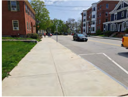
Improved sidewalks along Front Street
