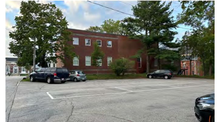
Municipal lots lack consistent town-branding and essential details indicating lot name, hours of operation, etc. (Source: Stantec Field Inventories)
