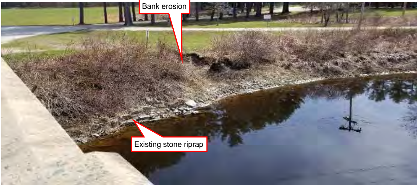
Photo No. 3 Description: Photo Date: 4/24/2018 Upstream right river bank
