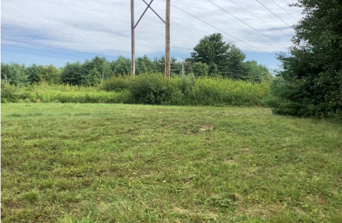
Photo 1. View northeast at existing Structure 177 to be replaced within the 300 foot shoreland buffer of the Little River in Exeter. Structure 177 is located immediately north (downslope) of Route 101 WB.
