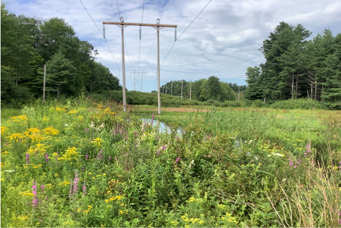
Photo 1. View southwest at existing Structure 176 to be removed from Wetland W31 and the associated floodplain and relocated within an upland area approximately 200 feet back (north) closer to Epping Road. Photo depicts approximate locations of temporary impact associated with timber matting.
