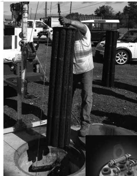
Cartridge Removal & Lifting Device
