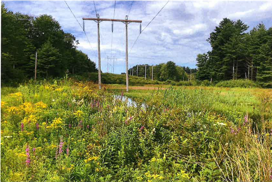
Photo 1. View southwest at existing Structure 176 to be removed from Wetland W31 and the associated floodplain and relocated within an upland area approximately 200 feet back (north) closer to Epping Road. Photo depicts approximate locations of temporary impact associated with timber matting.
