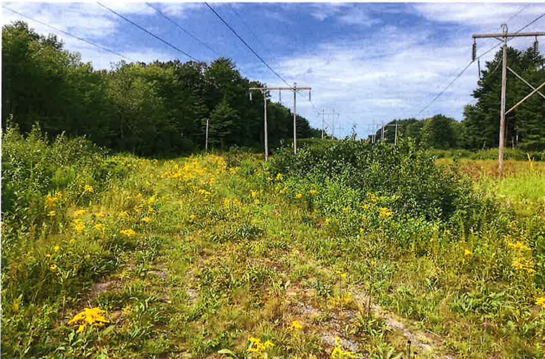
Photo 2. View southwest at general location of the proposed work pad required for the installation of new Structure 176. A portion of the work pad intersects the 300 foot shoreland buffer of the Little River. Existing Structure 176 (depicted in photo background, left) will be removed.
