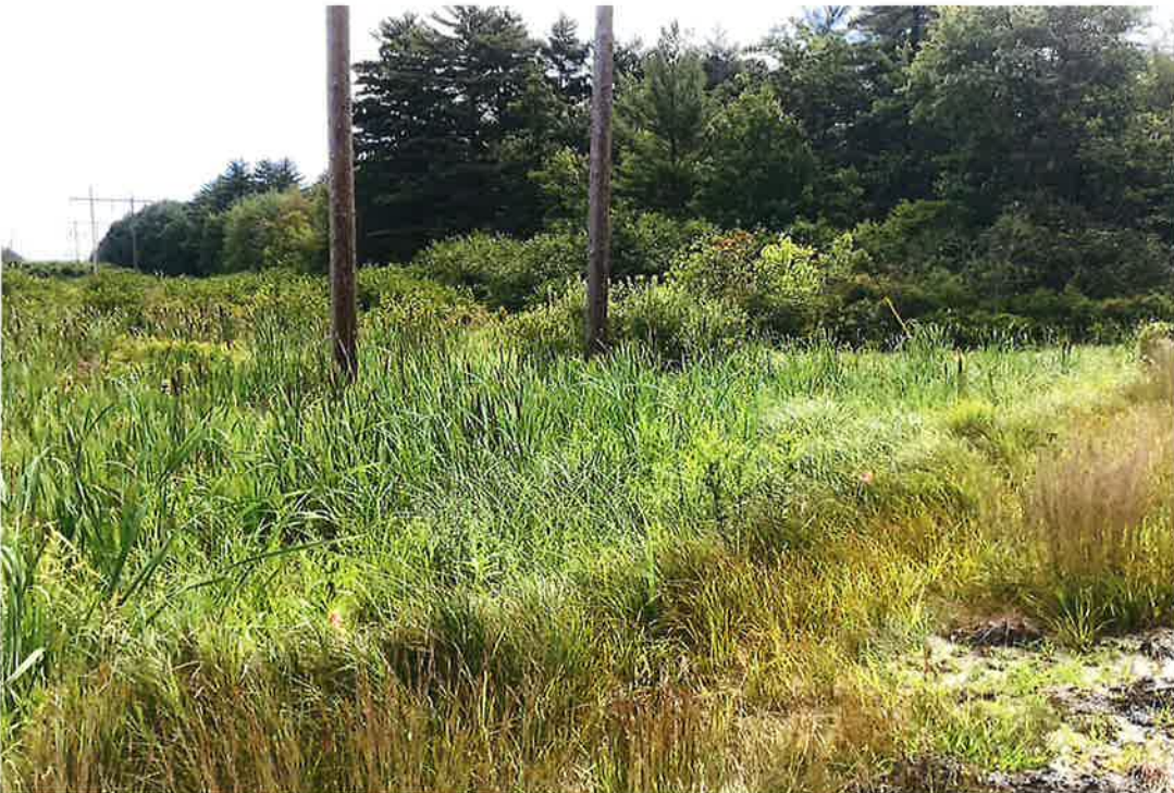
Photo 4. View northeast at existing Structure 175 to be replaced as part of the proposed project. Photo depicts the approximate location of a timber mat work pad (and resultant temporary impacts to Wetland W33) required to complete the structure replacement.
