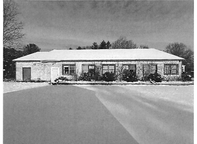
Description: Church, south side.
