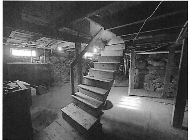
Description: Basement of residential house.
