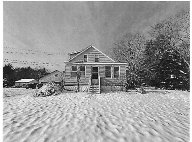
Description: Residential house, east side.
