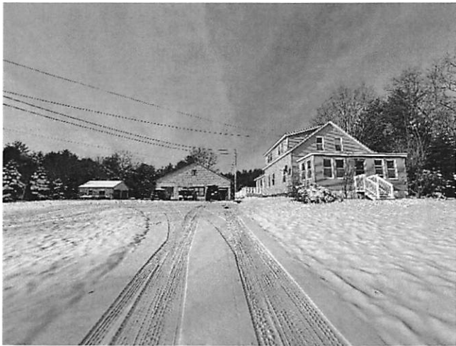
Description: Target Property at 50 Newfield's Road, Exeter, NH
