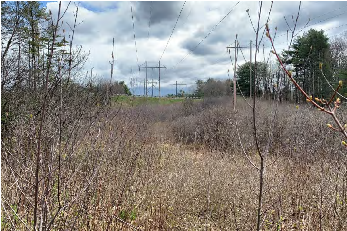
Photo 4. View east at location of proposed timber mat access road through Wetland EW-2 (NHDES Prime Wetland) required in order to access and replace Structure 200 (depicted in photo background).
