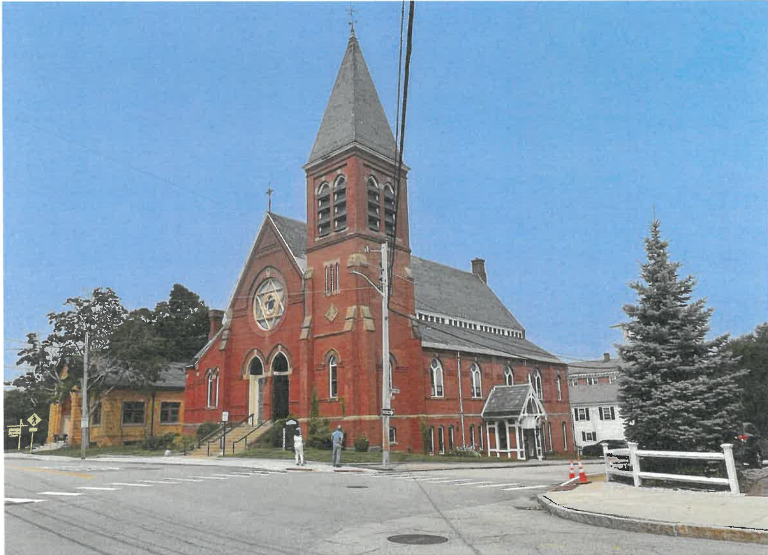
Existing Photo From Southwest Corner
