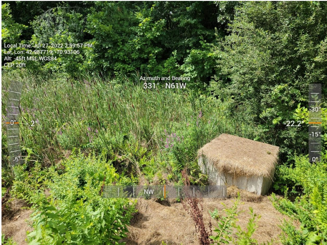
Photo: 5 – Detention-pond and outflow structure
