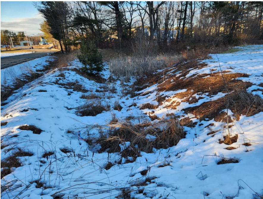
Image captures existing mad made wetland off site which captures and treats site runoff.
