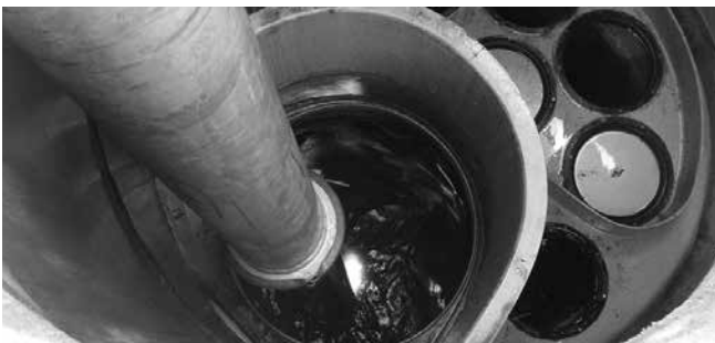
Vacuuming Sump Through MAW
