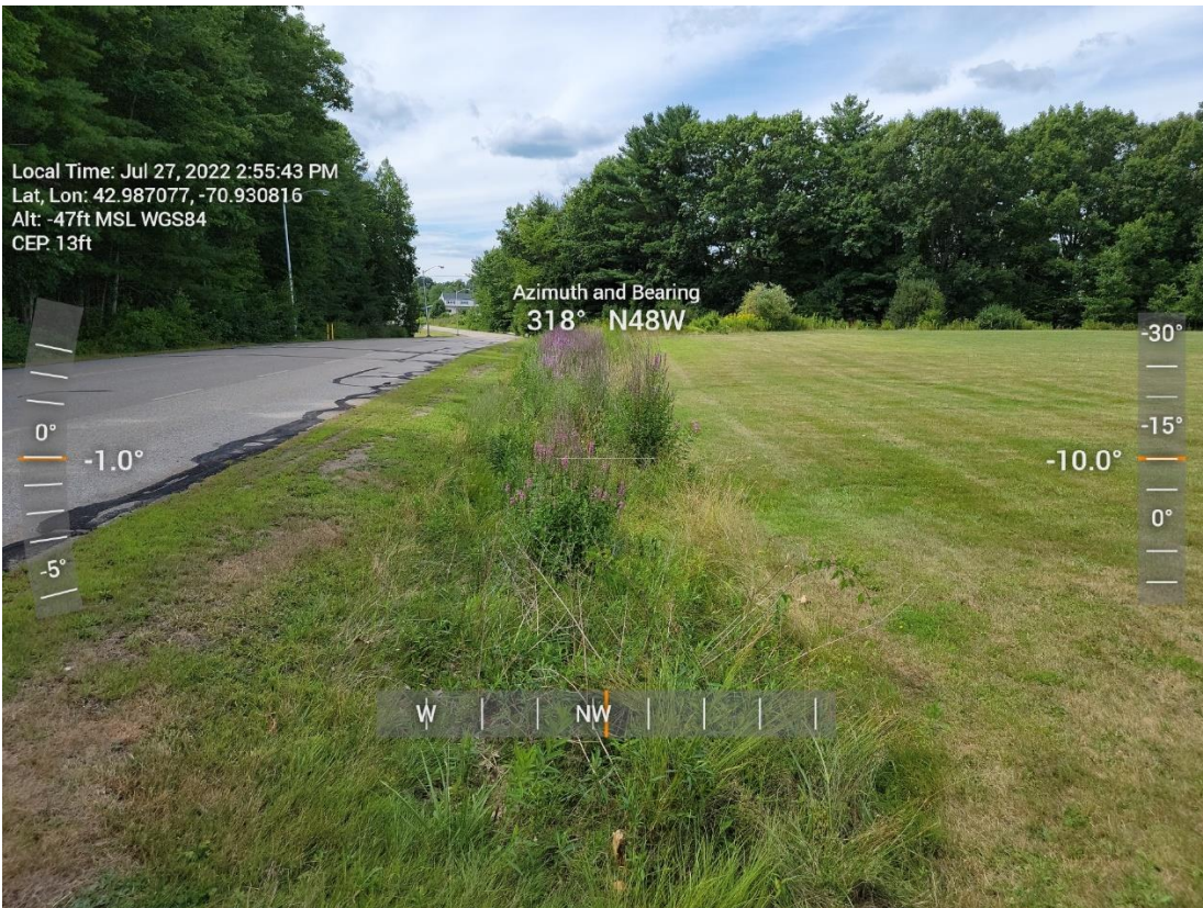
Photo: 8 – Roadside ditch diverting sheet flow to the detention-pond.
