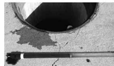
Inspection Utilizing Sediment Probe
