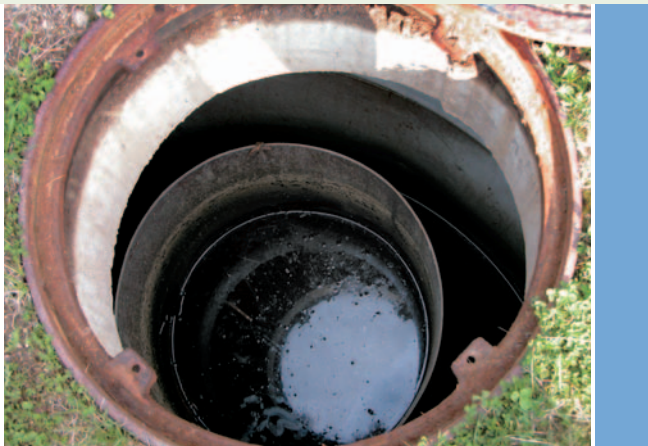
The CDS unit has a filter screen that can be sized by the vendor to accommodate a range of particle sizes.
