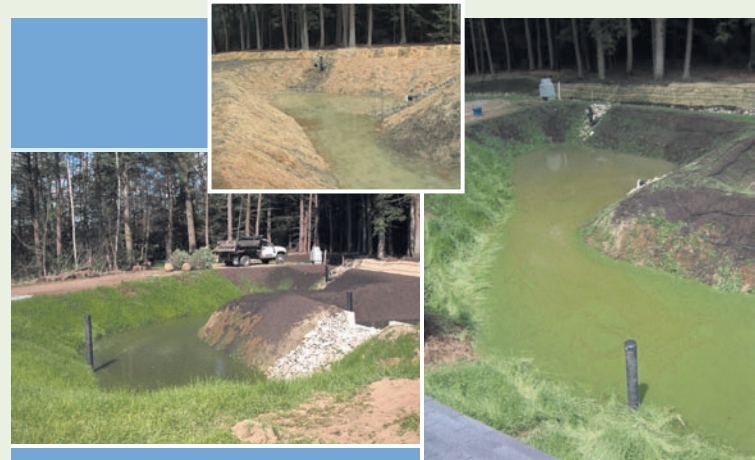
A pond's [left] water quality performance is a function of storage volume and retention time. Erosion control matting [center] protects slopes with a grade of 2:1 or steeper. Green water [right] is a sign of eutrophication, a water quality issue associated with retention ponds.
