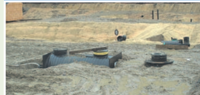
The Aqua-Swirl [right] uses a vortex and baffle to remove sediment, oils, and trash. The Aqua-Filter [top left] uses a physical and chemical process to remove sediment and other pollutants. These units can be used independently, or combined as a system [bottom left].
