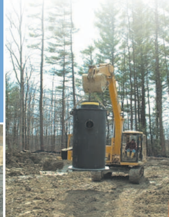
The Aqua-Swirl [right] uses a vortex and baffle to remove sediment, oils, and trash. The Aqua-Filter [top left] uses a physical and chemical process to remove sediment and other pollutants. These units can be used independently, or combined as a system [bottom left].
