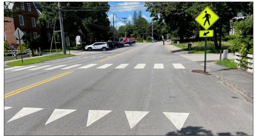
High visibility crosswalk markings installed on Front Street in 2023
