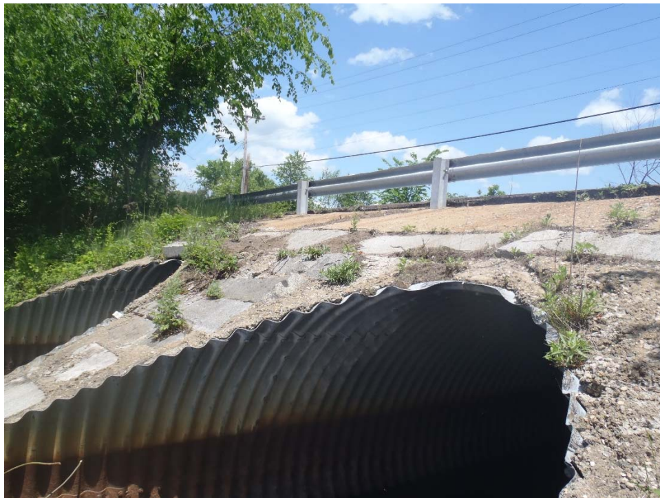
Typical stone and cast-in-place concrete infill headwalls between arches
