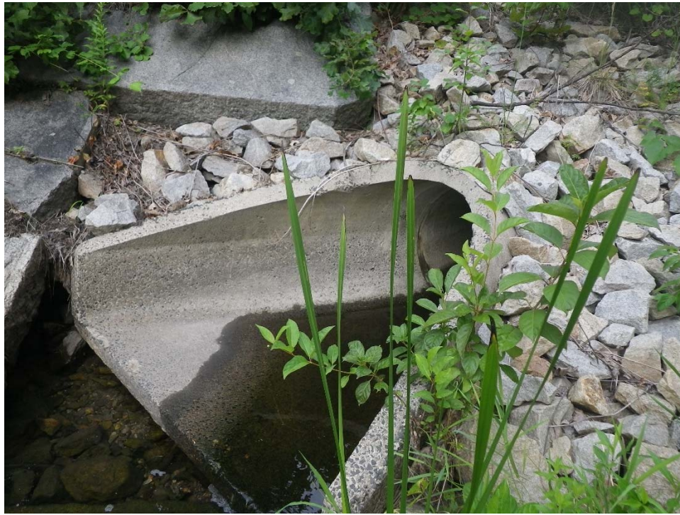
Concrete outlet structure near the north-east corner of the crossing
