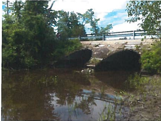
View of Linden Street culverts looking westerly.
