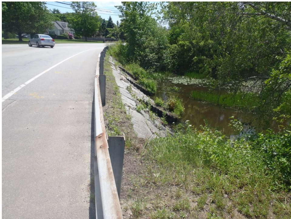
Typical dry-laid granite block headwalls
