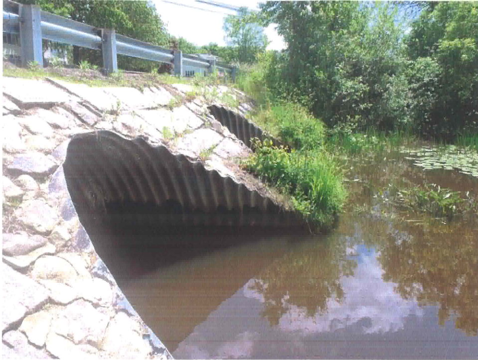
Typical headwall construction with granite and concrete
