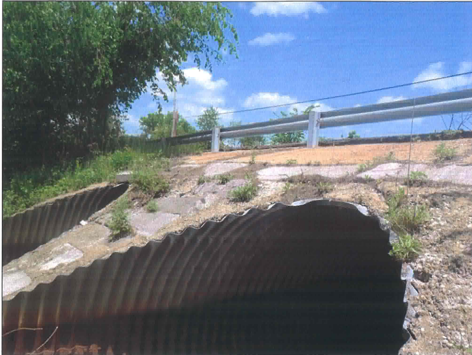
Typical headwall construction with granite and concrete infill
