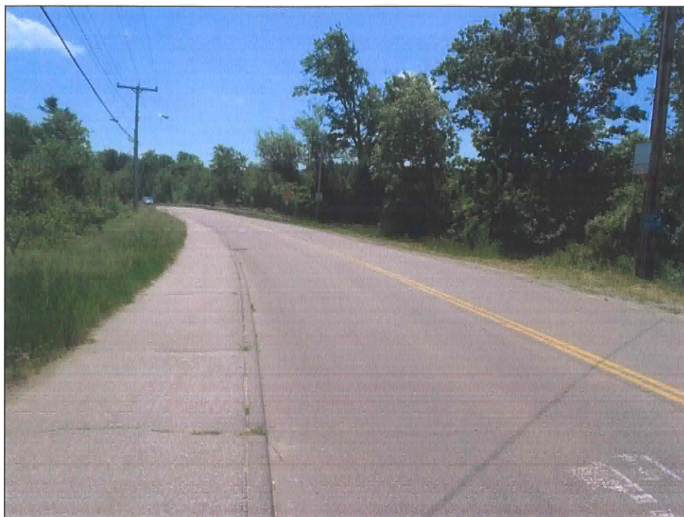
Linden Street north approach looking south (downstream is to the left)
