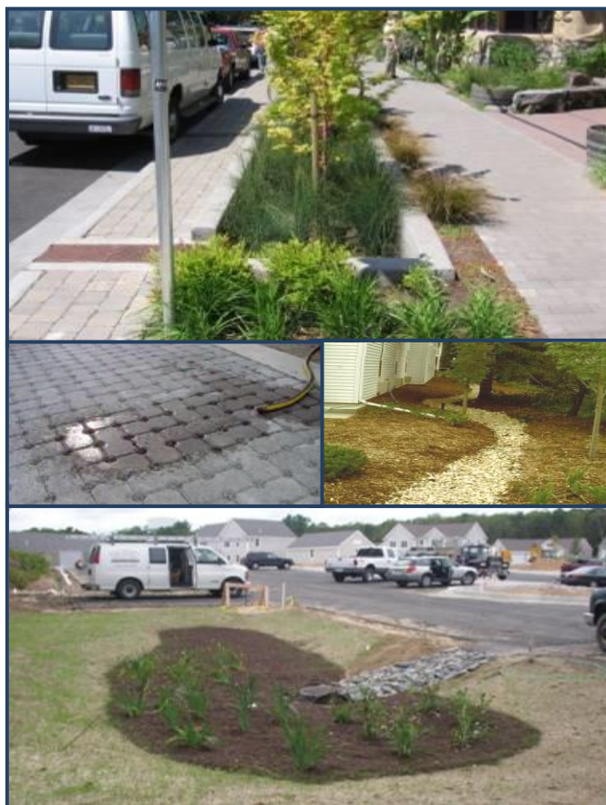
Figure 2. BMPs such as the bioretention, porous pavers, and infiltration trenches seen here are designed to provide water quality treatment and maximize runoff reduction through improved infiltration, evapotranspiration, and plant uptake. These are effective practices for reducing DCIA.
