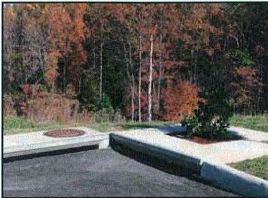
1. Inspection of Filterra and surrounding area
