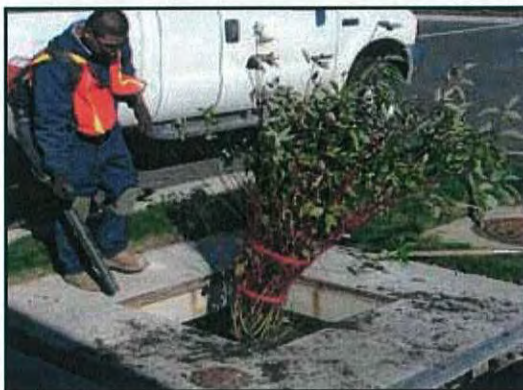
5. Clean area around Filterra
