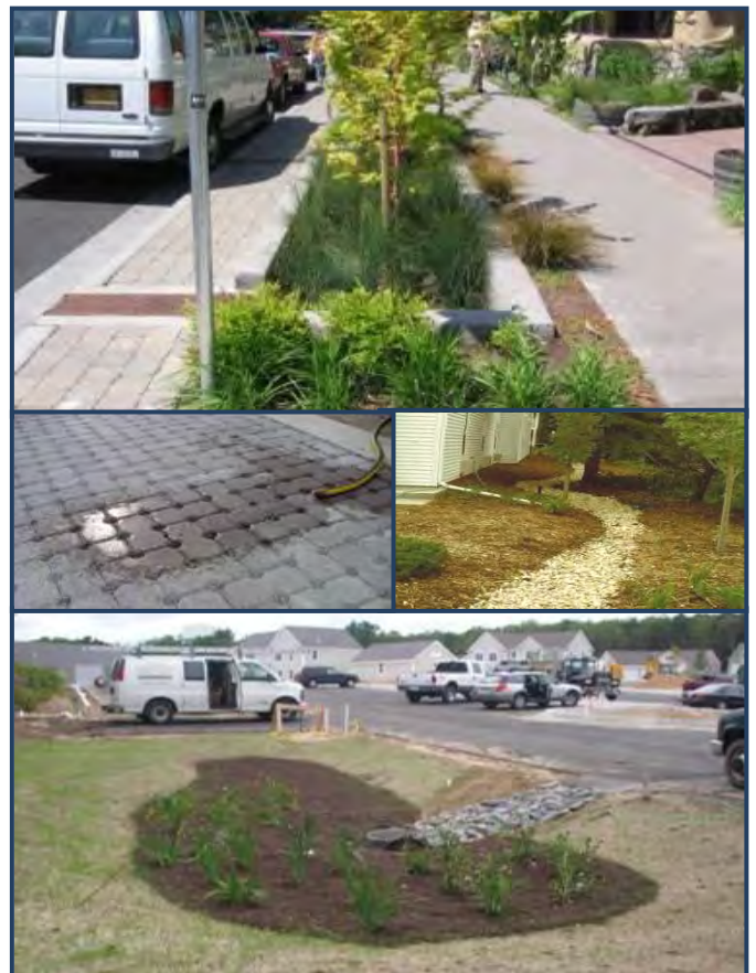
Figure 2. BMPs such as the bioretention, porous pavers, and infiltration trenches seen here are designed to provide water quality treatment and maximize runoff reduction through improved infiltration, evapotranspiration, and plant uptake. These are effective practices for reducing DCIA.
