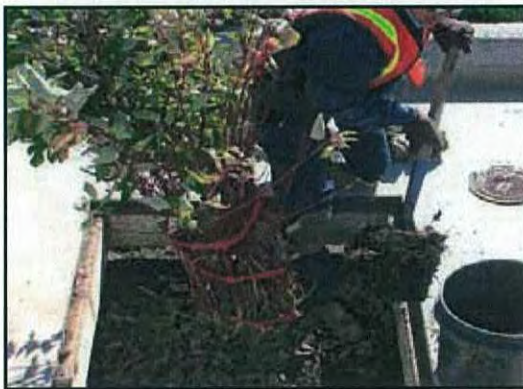
3. Removal of debris, trash and mulch
