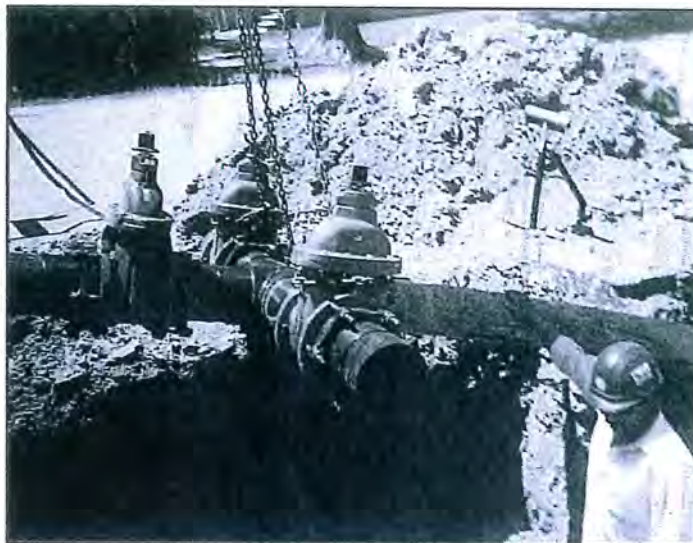
The project called for 97,000 feet of distribution lines, 108 fire hydrant assemblies, 804 service connections (not including schools) and more than 400 operating gate valves
