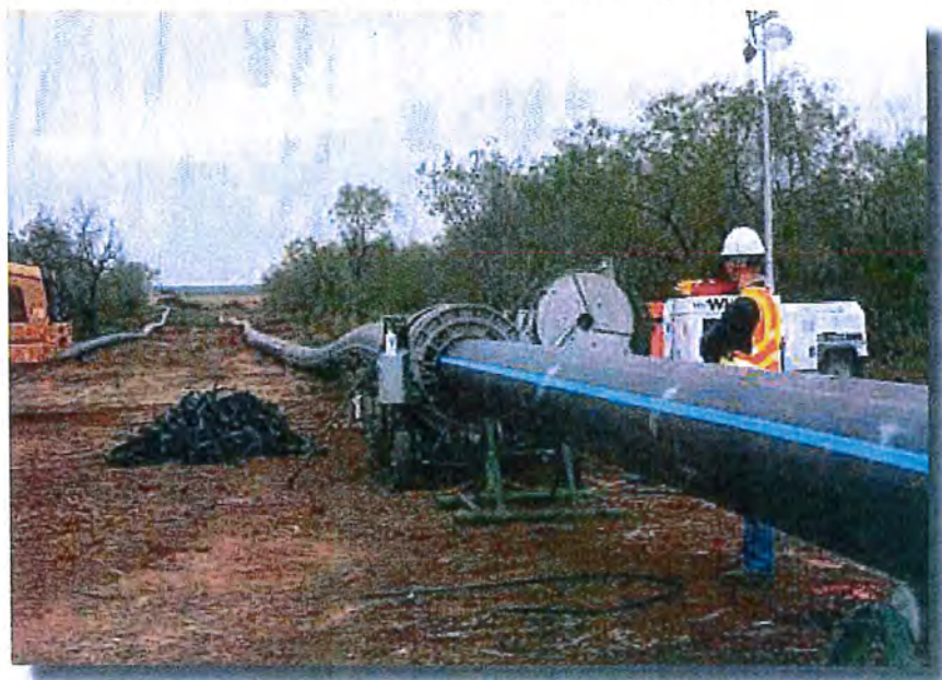
ISCO representative viewing a string of 24-inch DR 9 pipe on the SAWS project
