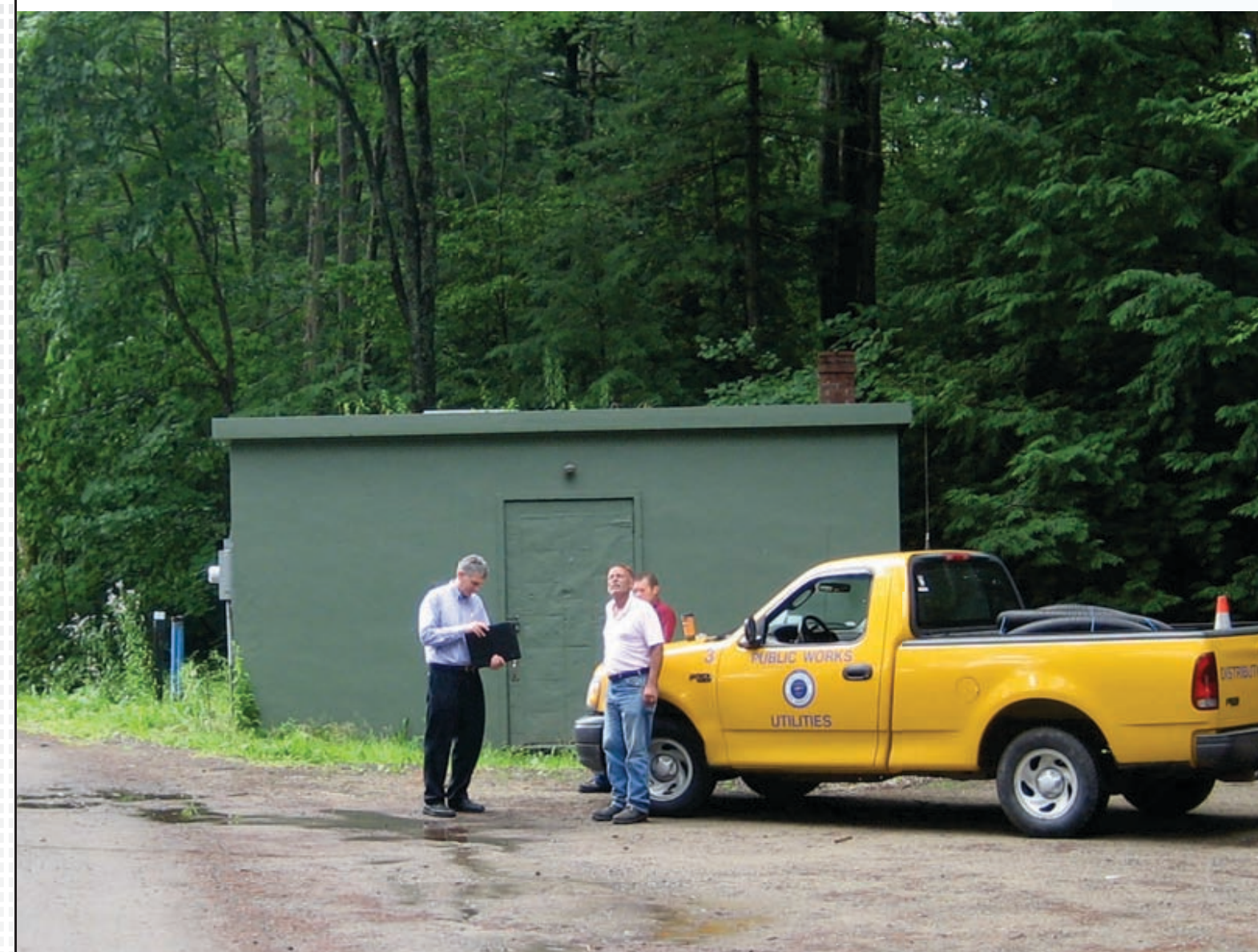
Existing Well Building
