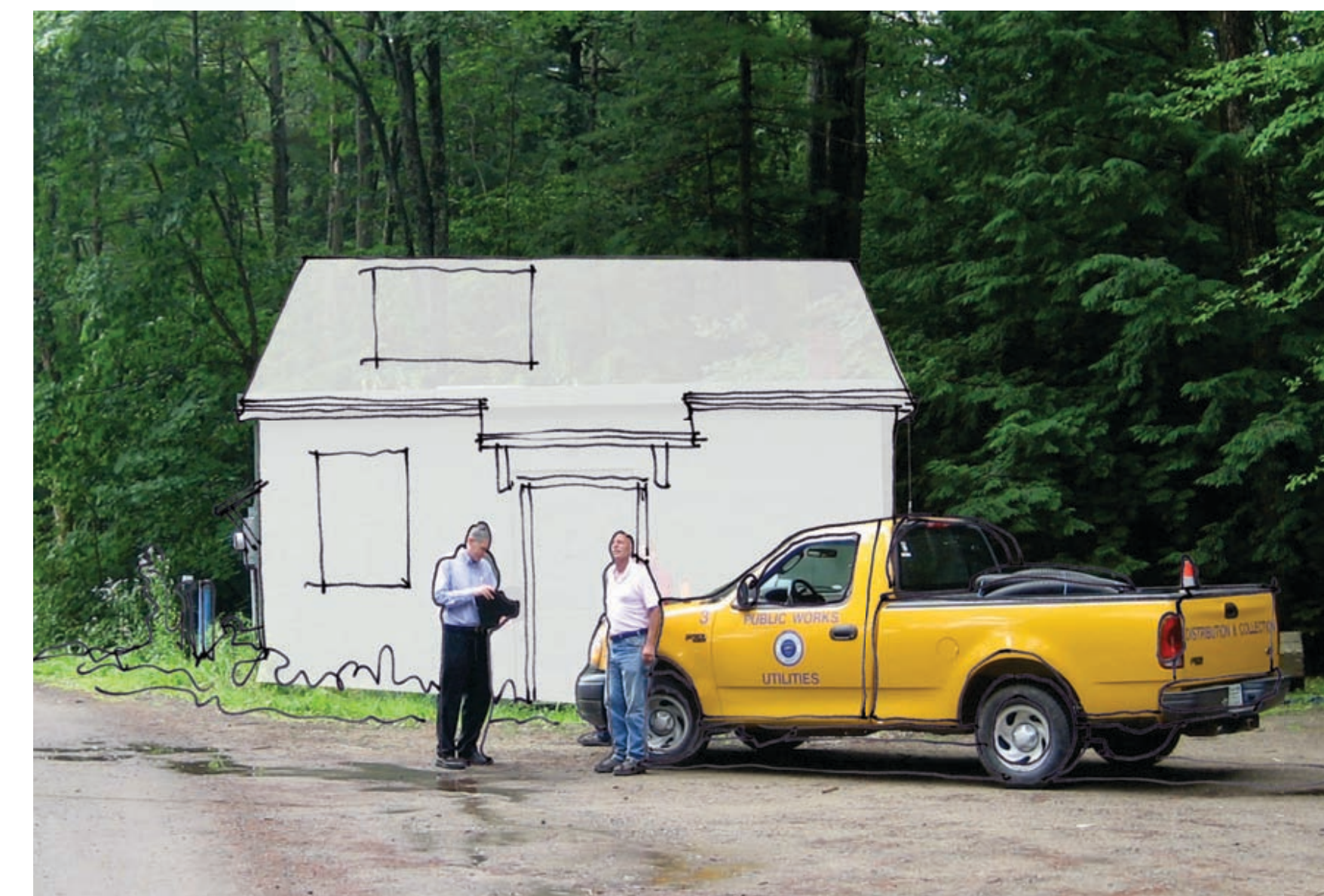
Renovated Well Building
