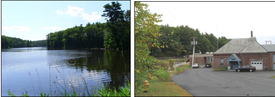
The Exeter Reservoir and Existing Surface Water Treatment Facility
