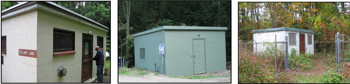
Existing Lary Lane and Gilman Park Wells – Stadium Well Prior to Rehabilitation
