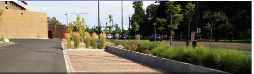
Permeable pavers are used in compact parking stalls, which have lower traffic volume than the driving lanes.
