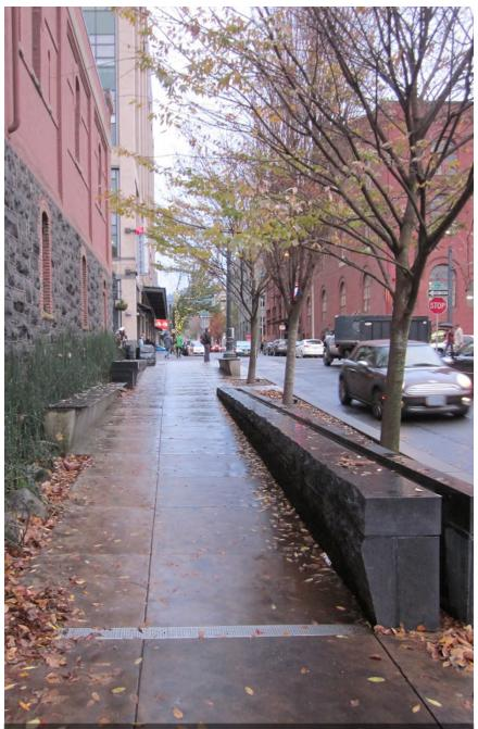
The low stone walls on either side of this sidewalk artfully funnel rainwater to a flow-through planter along the side of a building.
