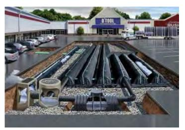
Figure 7. Subsurface infiltration at a commercial parking lot. (Credit: www.waterworld.com)
