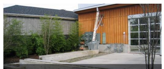
The concrete walls of this drywell offer seating around the perimeter of a courtyard, and an artful downspout creates a focal point.
