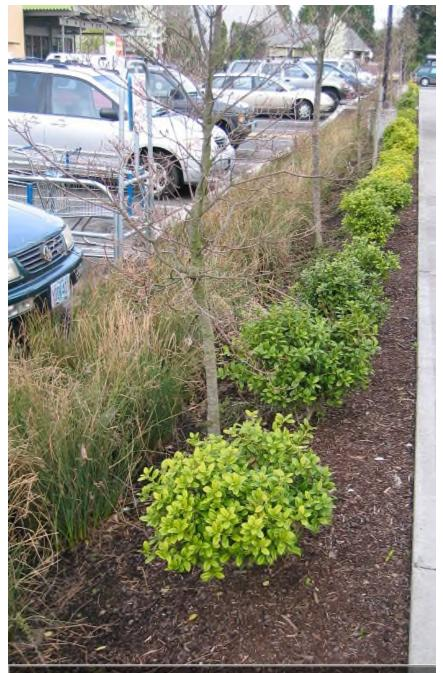
A bioretention area treats runoff from the parking surface and is planted with low-maintenance vegetation.
