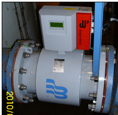
Photo of New Mag Meter at River Pumping Station and Testing the Meter in July 2010
