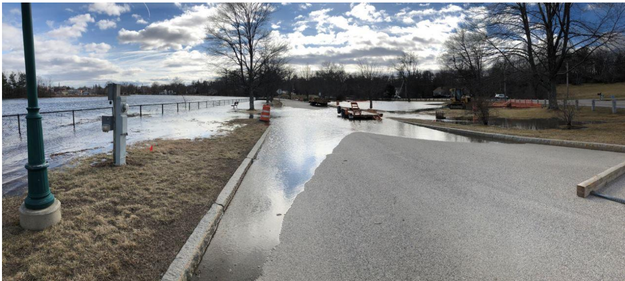
Figure 2: Flooding along Swasey Parkway from the Squamscott River during the March 2018 Noreaster
