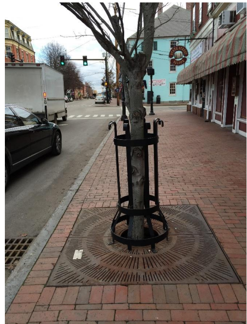
Figure 7: Tree Planter Combined with Catch Basin
