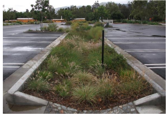
Figure 8: Parking Lot Bioretention
