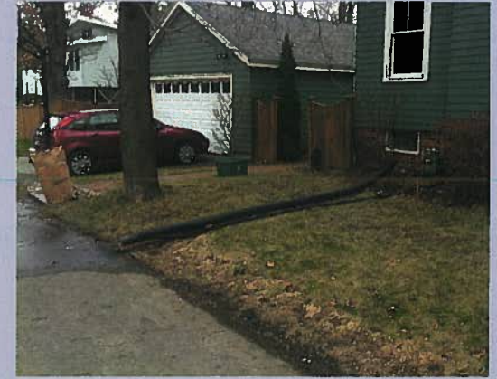
This can lead to icing and other maintenance issues
