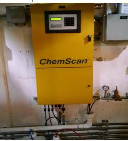
New Chemical Feed area at the Surface Water Treatment Plant which feeds an Ammonium Sulfate Solution into the Finished Water to generate Monochloramines for Disinfection, and the ChemScan analyzer that automatically monitors and controls the level of disinfectant in the Plant Output. This is duplicated at the Groundwater Facility...
