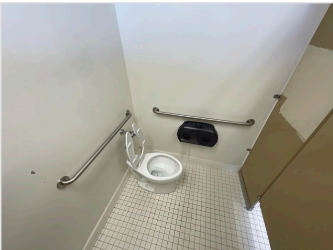
TOILET STALL OVERVIEW
