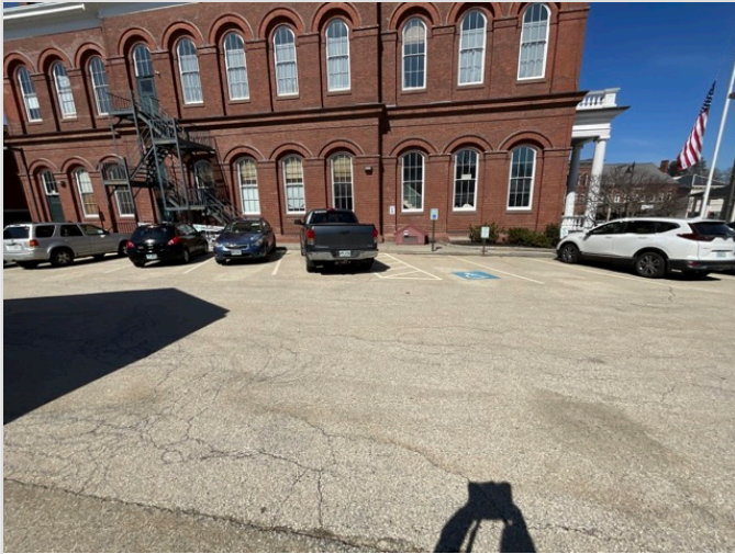
OVERVIEW OF ACCESSIBLE PARKING AREA
