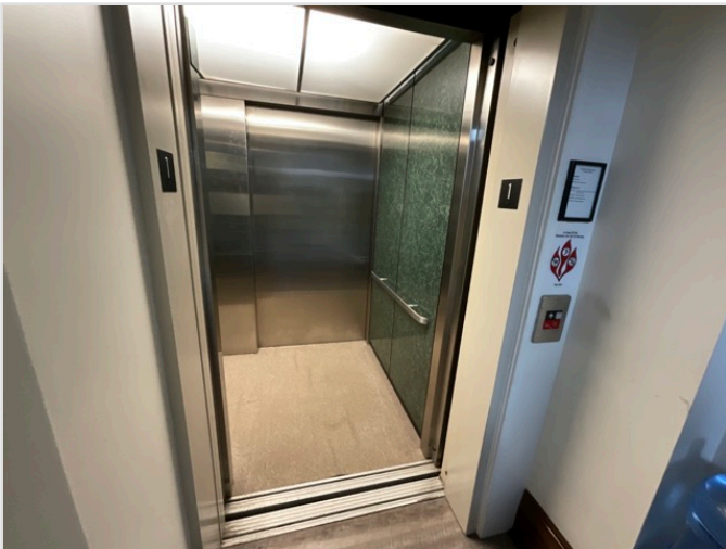
LOBBY LOOKING AT CABS (WITH DOORS OPEN)
