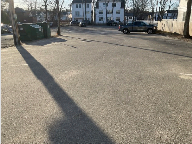
OVERVIEW OF ACCESSIBLE PARKING AREA
