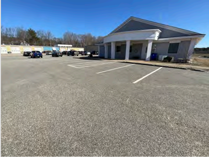
OVERVIEW OF ACCESSIBLE PARKING AREA
