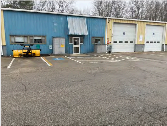
OVERVIEW OF ACCESSIBLE PARKING AREA
