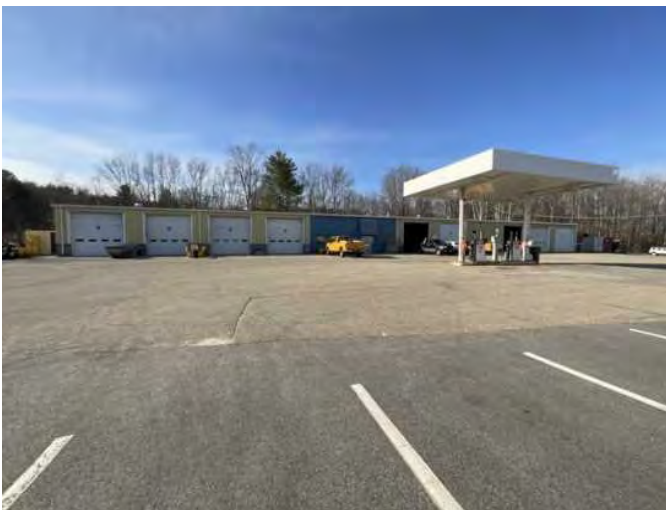
41 - GARAGE BAY WITH PUMPS
