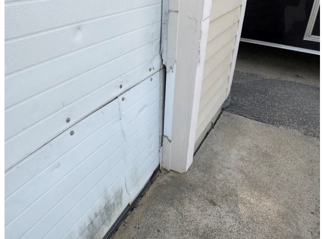
20 - DAMAGED WEATHSTRIPPING
