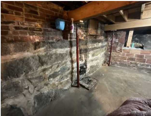
9 - JACK POST SUPPORTS
