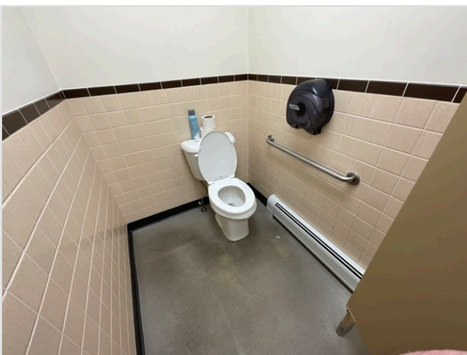
TOILET STALL OVERVIEW
