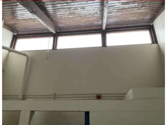
8 - CEILING STRUCTURE IN LOCKER ROOM
