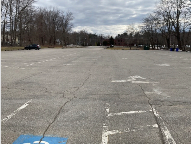
OVERVIEW OF ACCESSIBLE PARKING AREA
