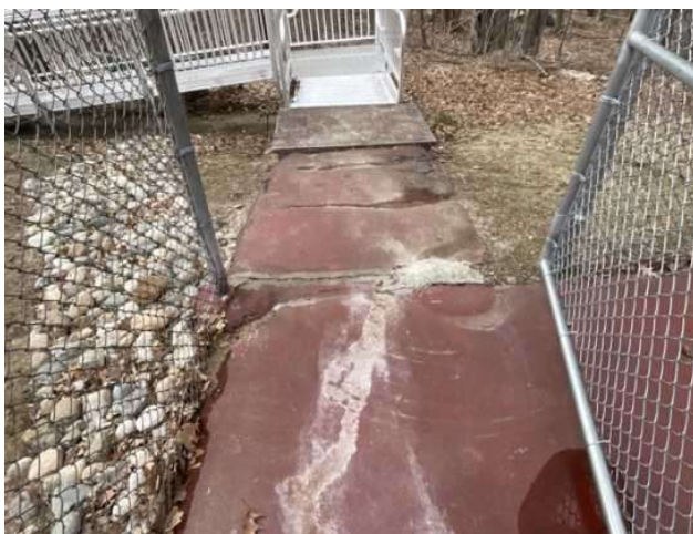
23 - RAMP SIDEWALK TO COURTS
