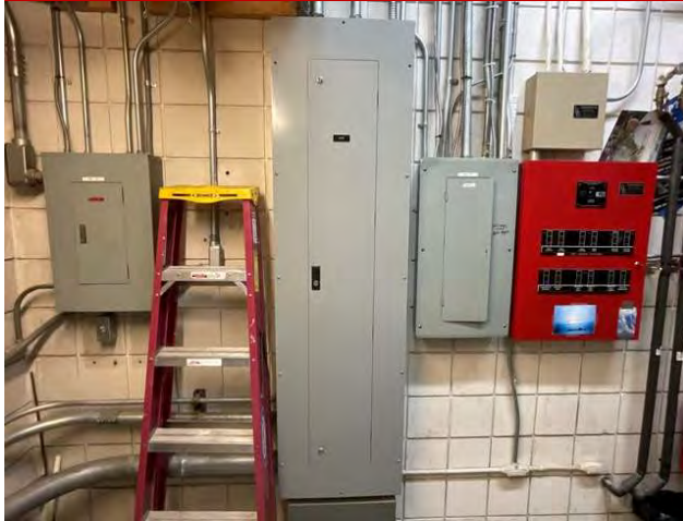
19 - LOAD CENTERS AND FIRE ALARM PANEL
