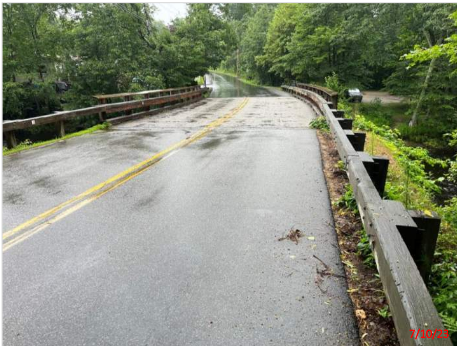
Photograph 2 – View of Linden Street Bridge Deck and Approach (Facing North)
