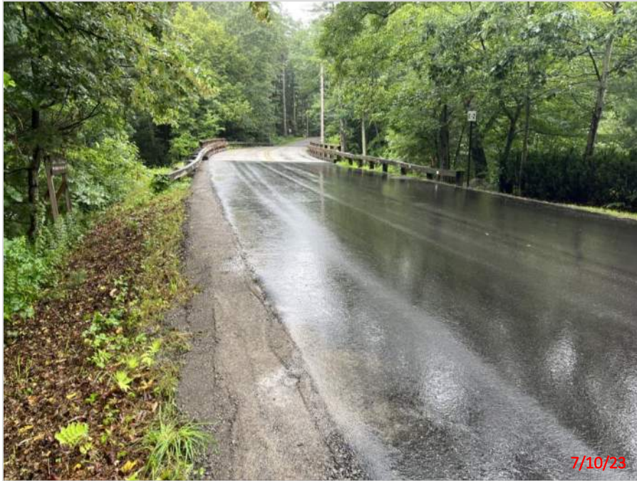
Photograph 3 – View of Linden Street Bridge Deck and Approach (Facing South)
