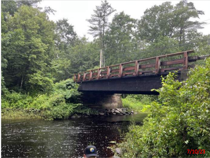
Photograph 1 – View of Linden Street Bridge over Exeter River (Facing Southwest)
