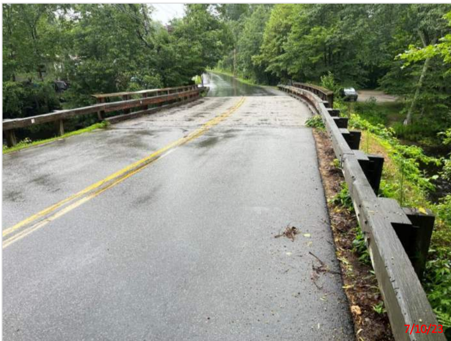
Photograph 4 – View of Linden Street Bridge Deck and Approach (Facing North)
