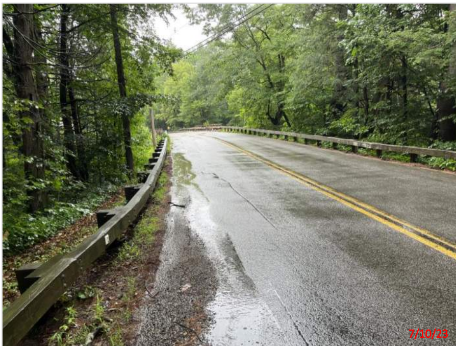
Photograph 4 – View of Linden Street Bridge Approach (Facing North)
