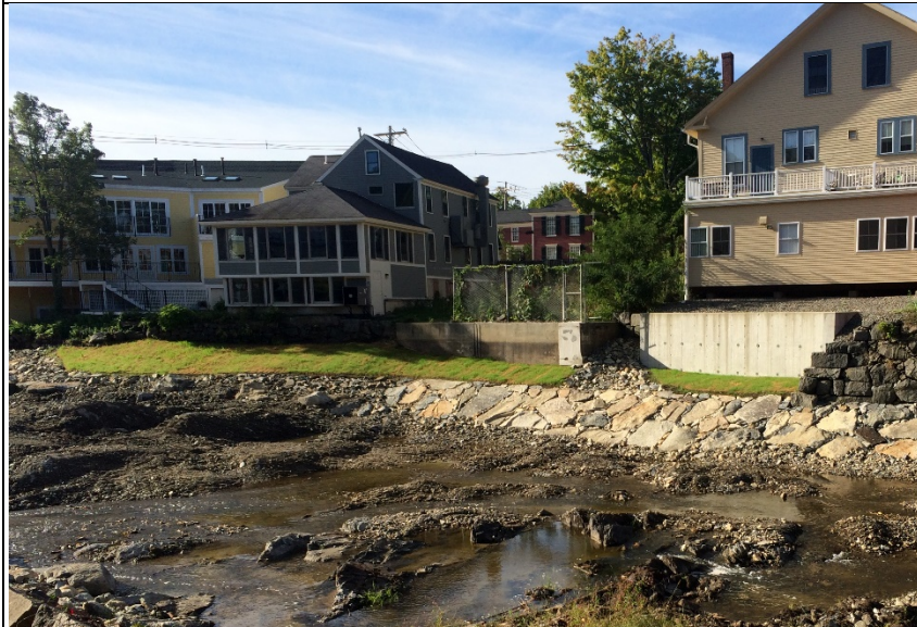
Immediately following construction, taken 9/16/2016
