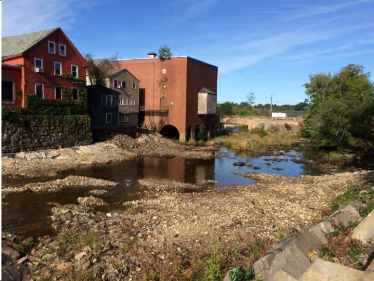
Description: Post-Construction, taken 9/21/2016
